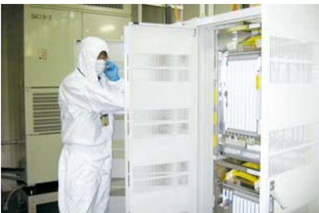
Replacing base station transmission lines (communications building in Tomiokamachi, Fukushima Prefecture)
