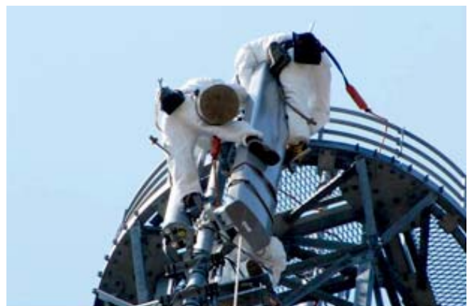
Installing high performance antenna (base station in Iwaki, Fukushima Prefecture)
