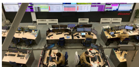
A network operation center monitoring facilities 24 hours a day, 365 days a year
