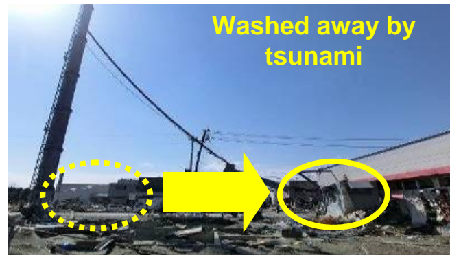
(2) Base station facility (Ishinomaki-Midori, Miyagi Pref.)
