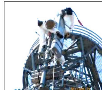
【Apr. 13, 2011】 Installation of high- performance antenna (Base station in Iwaki, Fukushima)
